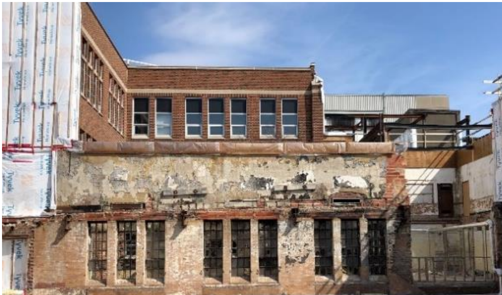
Post-fire view of dismantled east auditorium wall.
