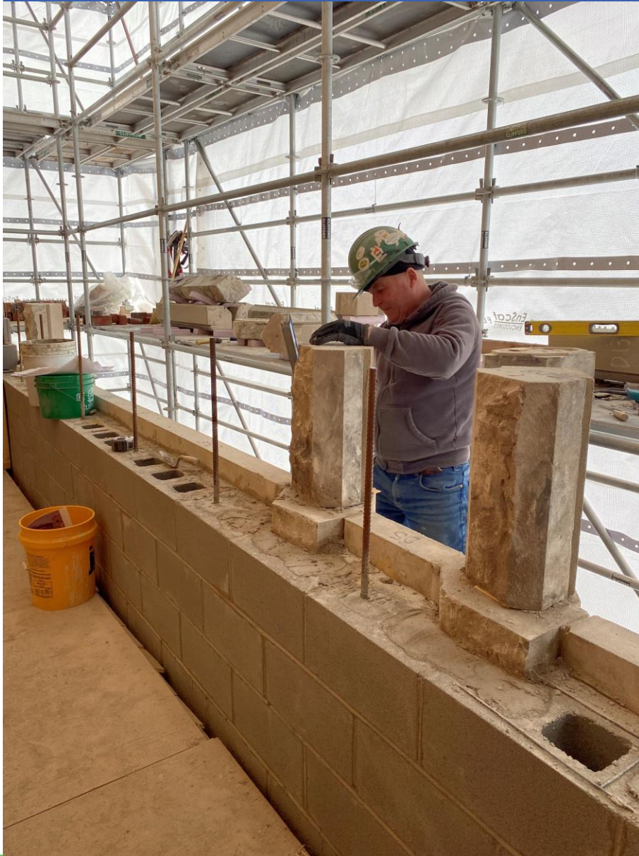
Restoration of the 1929 front façade east bay.
