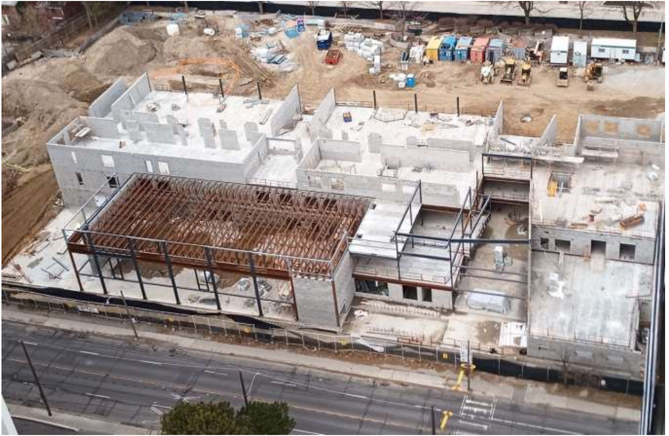
STATUS OF CONSTRUCTION – 5 April, 2020
